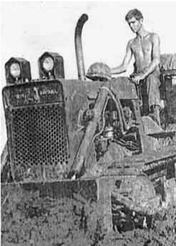
**MECHANIZED HELP** - A "mini-dozer" saves manhours at the 4th Division's Firebase Hooper in the Central Highlands by digging the larger bunker holes.
