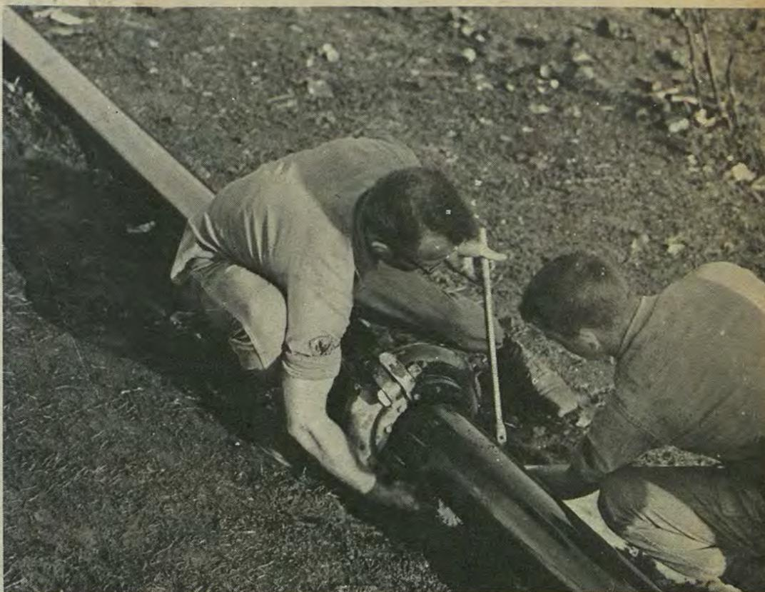
**HOLD IT TIGHT**—Two men from the 647th Quartermaster Company tighten a link in the six-inch pipe which runs along Highway 19 and pumps all the fuel from An Khe to Pleiku.
