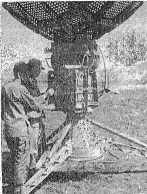
**CHECKING THE WEATHER**—Staff Sergeant Richard Roberts (Atkinson, Neb.), left, and Specialist 5 James Kelly (Klamath Falls, Ore.) of the meteorological section check out the Rawin Set (radio receiver) prior to sending a transmitter aloft to check weather conditions.
