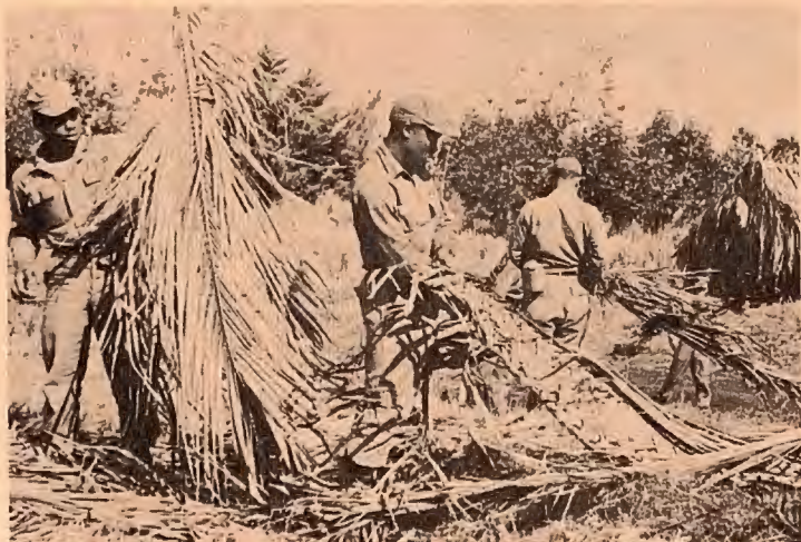
COVER HUTS — Members of the 65th Engr. Bn. used palm fronds to cover huts which they built for aggressor villages.
