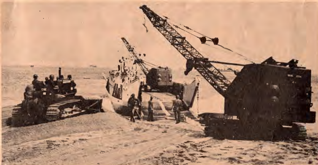
HEAVY EQUIPMENT - Marine cranes unload beach matting from a LCU (Landing Craft Utility) at Papohaku Beach.
