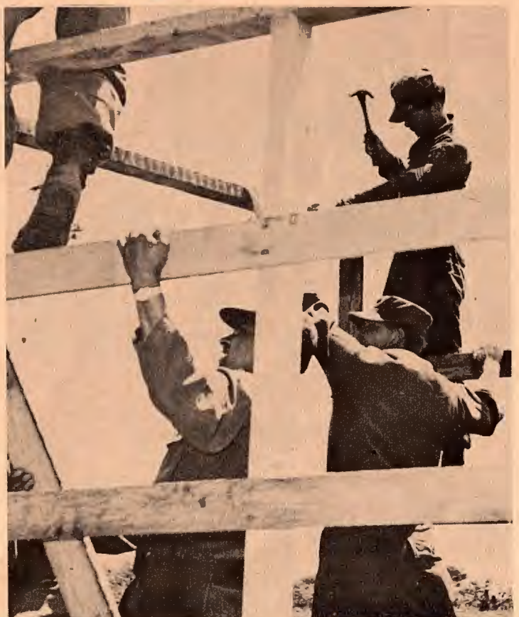
BUILD VILLAGE — Members of Co. C, 65th Engr. Bn., add boards to the frame of a hut in one of the three villages which they constructed for the aggressor "countries" of Bahka and Naka.
