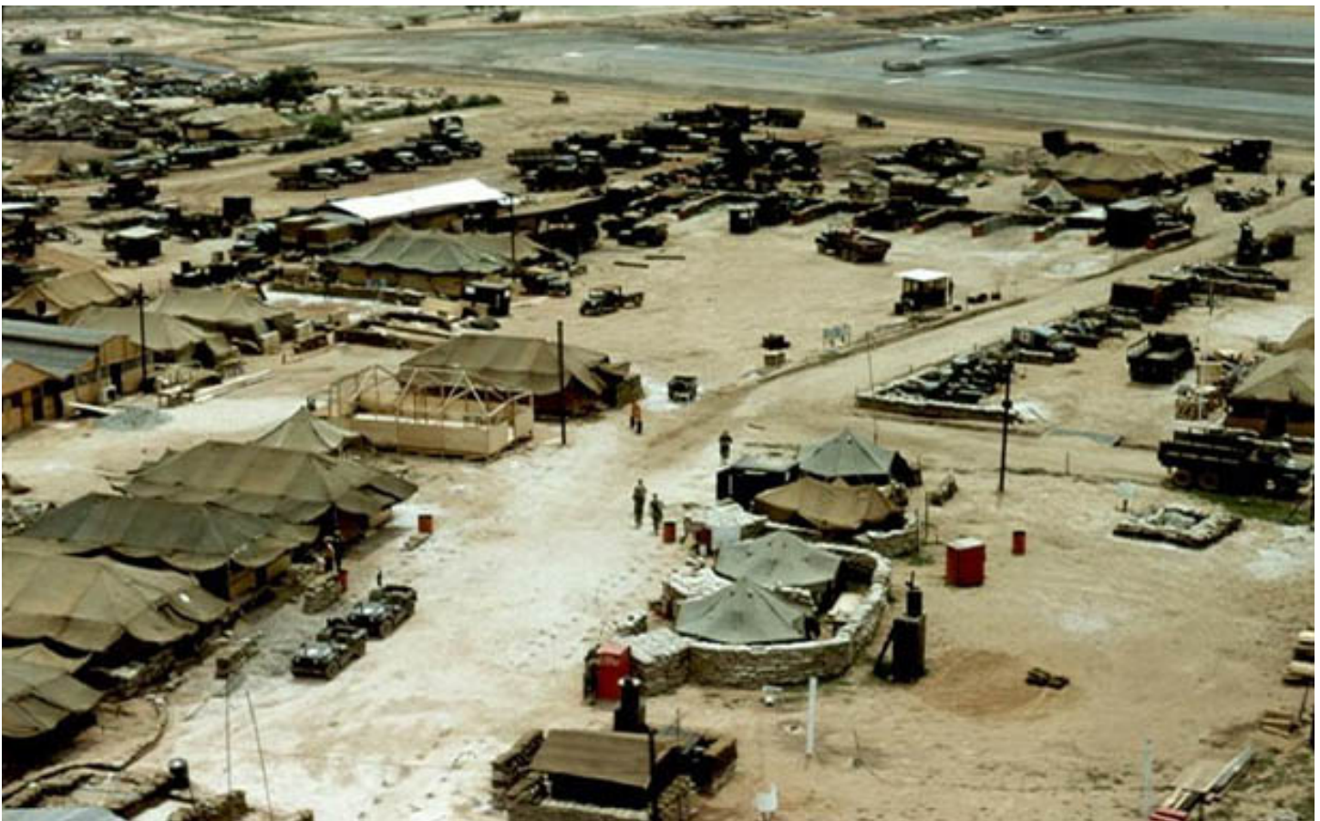
HQ, 3rd Brigade, 25th Inf Div, Duc Pho. LZ Montezuma, Spring, 1967. Construction of the Brigade Base Camp. Note runway at top and the use of wood, canvas & sandbags. Col James Shanahan, Commanding. Photo by Dennis Dauphin 1/9 th Arty
